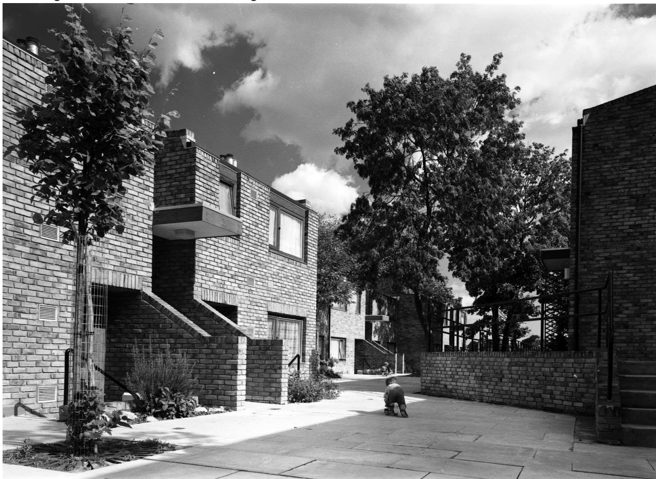
When Cressingham Gardens shortly after construction
