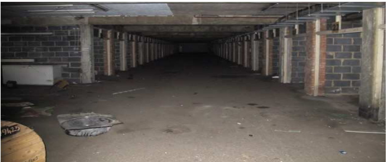
Parkhurst Road - garage space interior pre development
