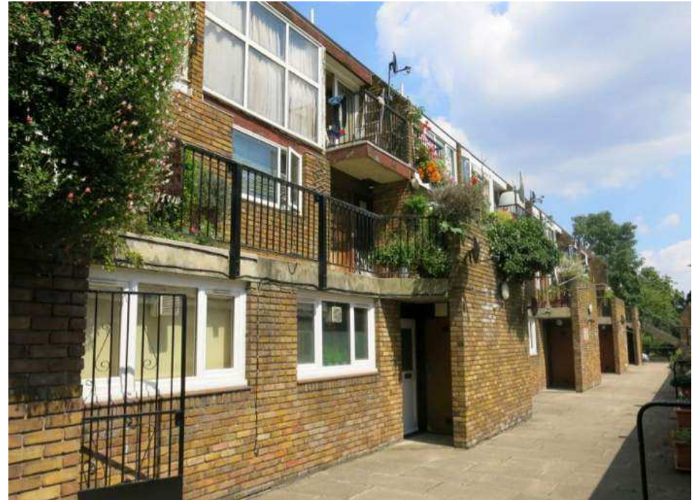
Village-like design using pedestrianised streets, high level balconies and maximising day lighting to create a safe community feel.
