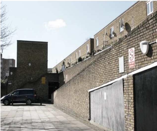
Parkhurst Road - Rear facade before
