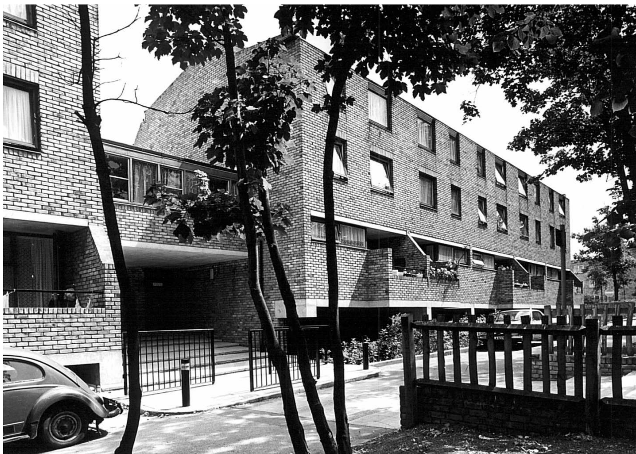
CGE immediately after build
