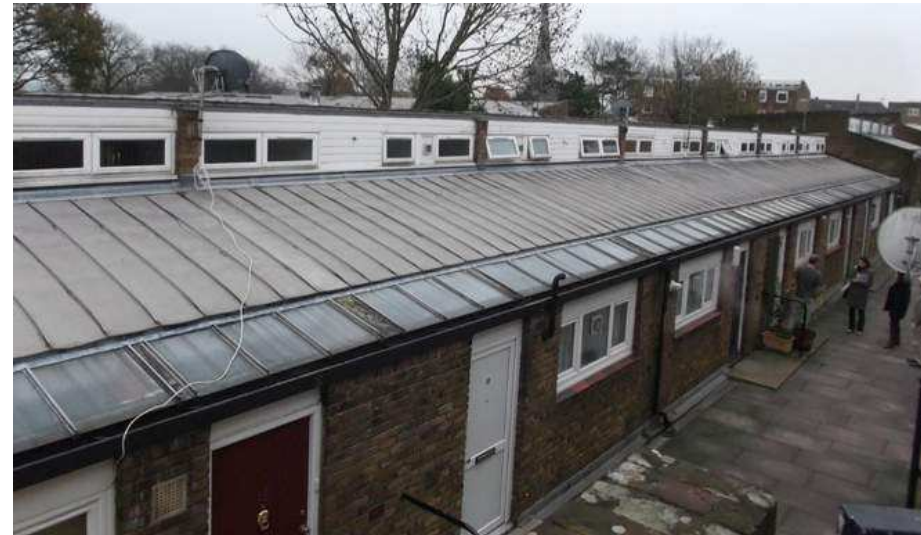
Existing roofs of Cressingham Gardens are predominantly low-rise zinc clad roofs.
