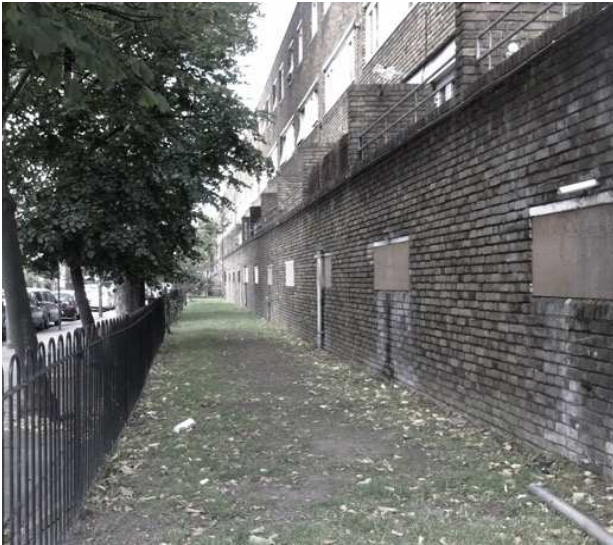
Parkhurst Road - Front facade before
