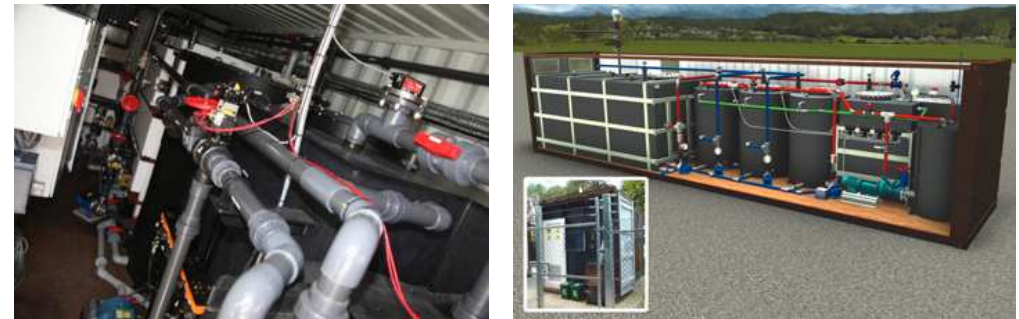
Anaerobic digester plant – compact installation
