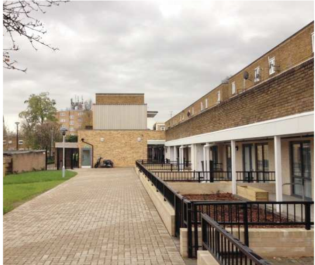
Parkhurst Road - Rear facade after
