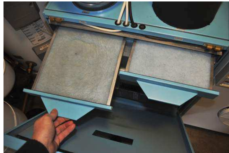
Intake air is filtered inside MVHR ensuring constant supply of fresh air
