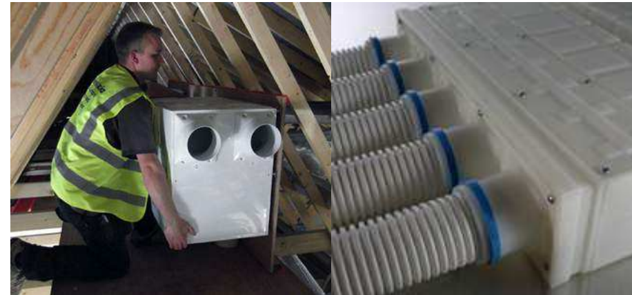
MVHR unit comes in different shapes and sizes to suit installation type (ceiling/ wall mounted, external/ internal), size of the dwelling and system requirements. The duct work is also
