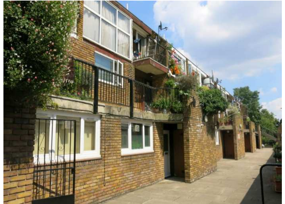
Village-like design using pedestrianised streets, high level balconies and maximising day lighting to create a safe community feel.
