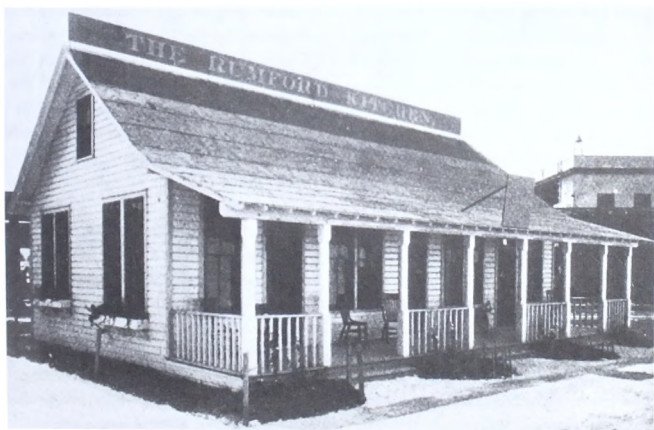
8.9 The Rumford Kitchen, an exhibit set up by Ellen Swallow Richards and Mary Hinman Abel for the World's Columbian Exposition, 1893, on the exterior a small, single-family clapboard house with a broad front porch
