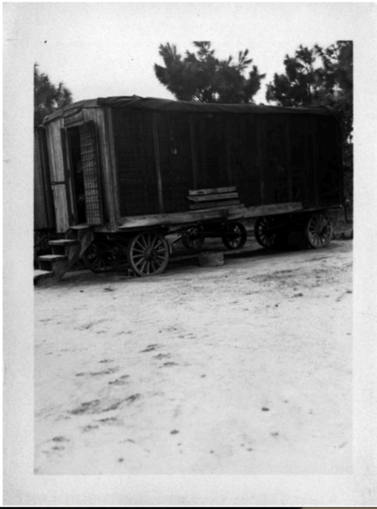
Figure 1.4. "The Cage: where convicts are herded like beasts of the jungle. The pan under it is the toilet receptacle. The stench from it hangs like a pall over the whole area" John Spivak, Georgia N_____, 1932.
