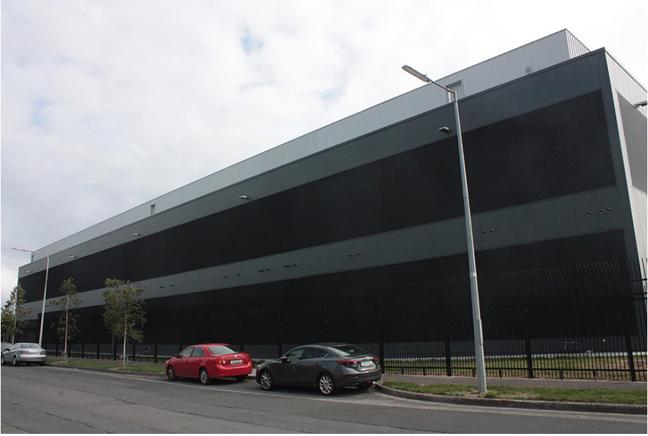
Fig. 4. Paul O' Neill, Side view of AWS data center on Greenhills Road, Tallaght, Dublin 24, 2018
