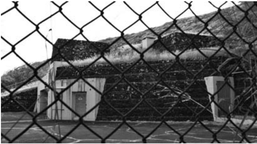
FIGURE 3.5. Hanauma Bay cable station, O'ahu, Hawai'i.
