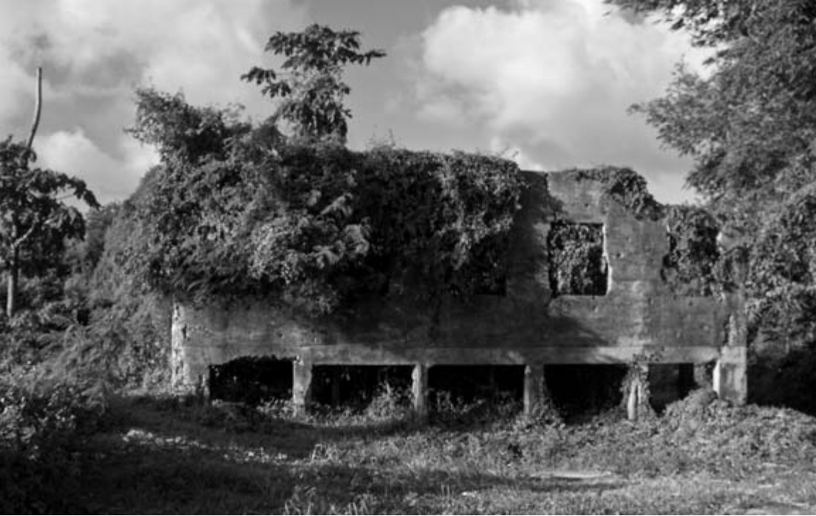
FIGURE 3.8. Ruins of Sumay cable station, Guam.
