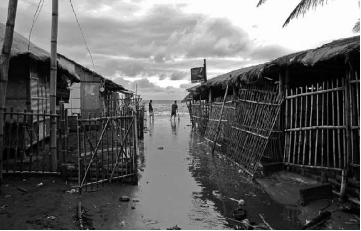
FIGURE 4.8. Nasugbu cable landing, the Philippines.
