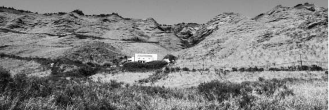
FIGURE 3.1. Keawa'ula cable station, O'ahu, Hawai'i.
