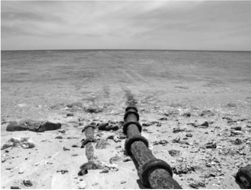
FIGURE 2.4. A cable conduit extends out to sea at Gun Beach, Guam.
